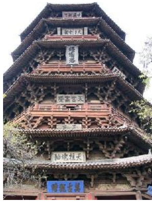
Detail of the dougong supports of the Sakyamuni Pagoda.
