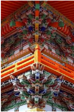
An example of dougong, a structural support of interlocking wooden brackets.
